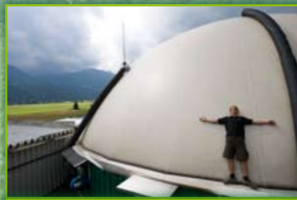
Biogas plant Würmlach
