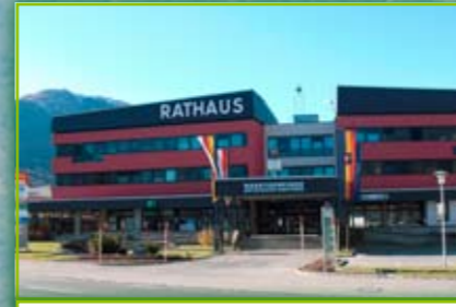
Energy information point City Hall
